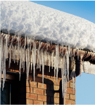
Ice dams form when heat escapes from your attic or the interior of your home and melts snow on your roof.
